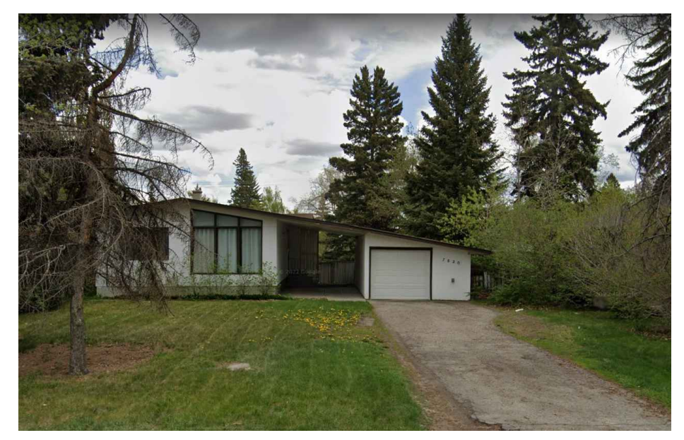
VIEW 2 - NW CORNER
